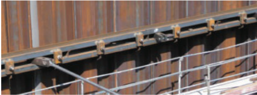
Convention Centre Bridge-Piling, Melbourne,Australia
